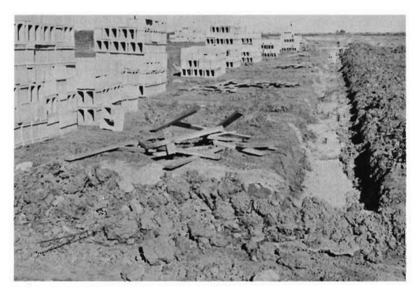
Excavation is completed and the foundation is poured. The concrete blocks are piled high in preparation of the task ahead.
